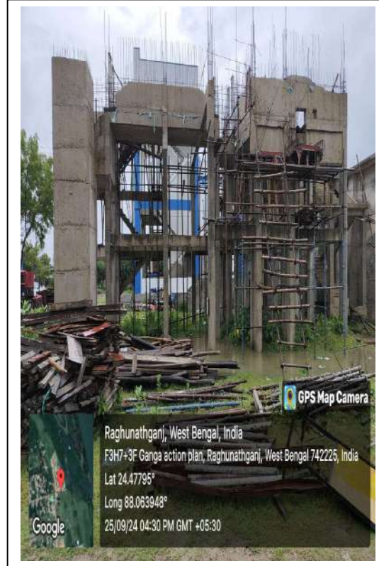
RAGHUNATHGUNJ STP SITE
